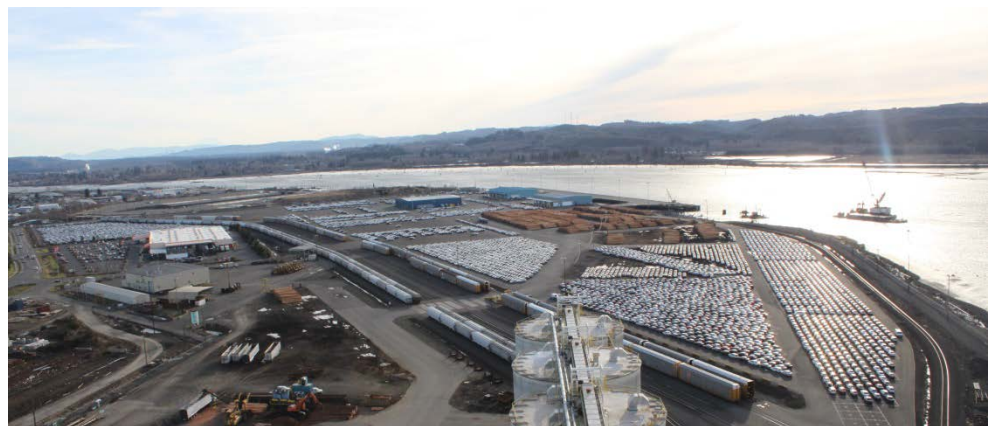
Road, rail, docks and the navigation channel are critical infrastructure that the Port's marine terminal tenants rely on to ensure their products are safely and efficiently connected to markets here in the US and throughout the globe.
